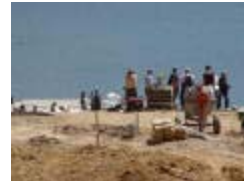
Tons of work to be done!!
